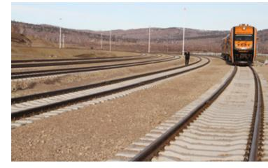
compatible with Chinese rails and all rails going North needs to be compatible with Russian rails. Moreover, there needs to be four tracks at the meeting point of those rails so trains can pass freely.
